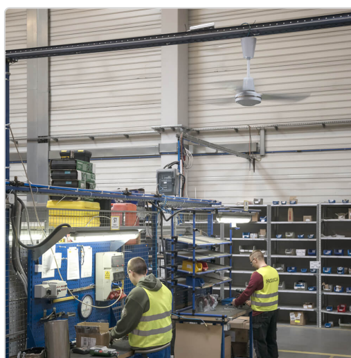
Master E destratifier workshop
